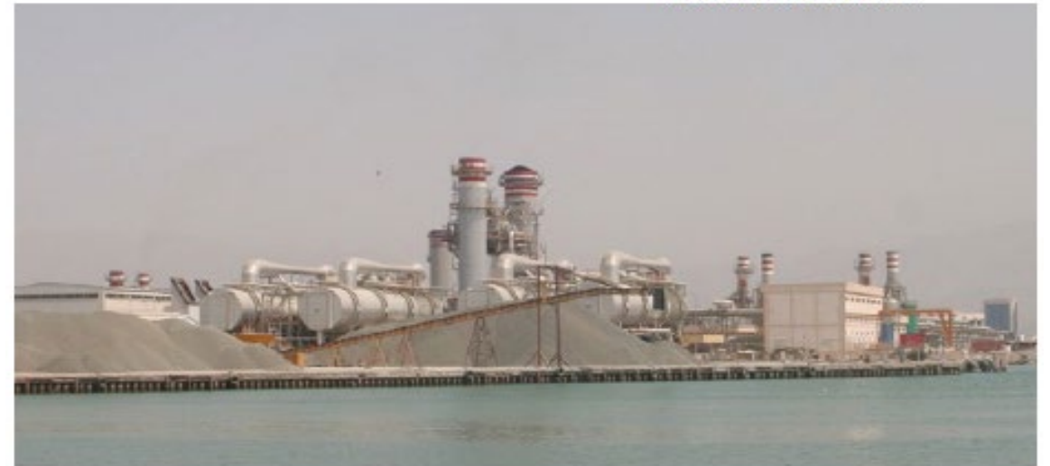
Fig. 2.4.9. A seawater desalination plant in the United Arab Emirates.
